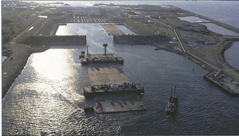
**Figure 10-5 Towing of a tunnel element mounted with immersion pontoons from a production facility.**
