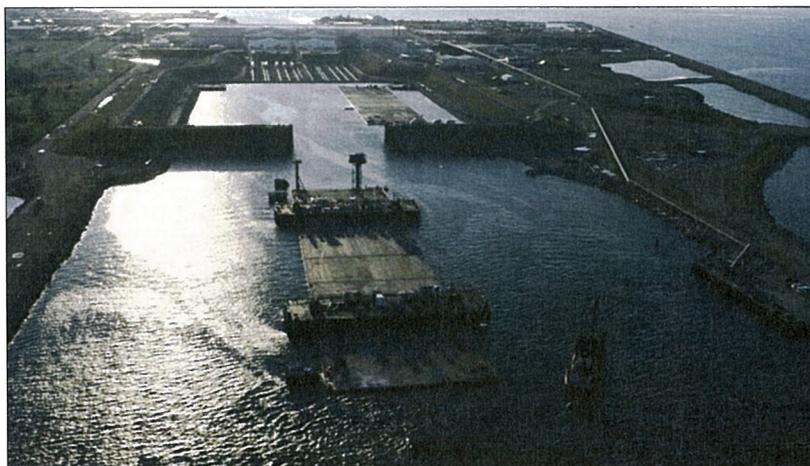
**Figure 11-5 Towing of a tunnel element mounted with immersion pontoons from a production facility.**
